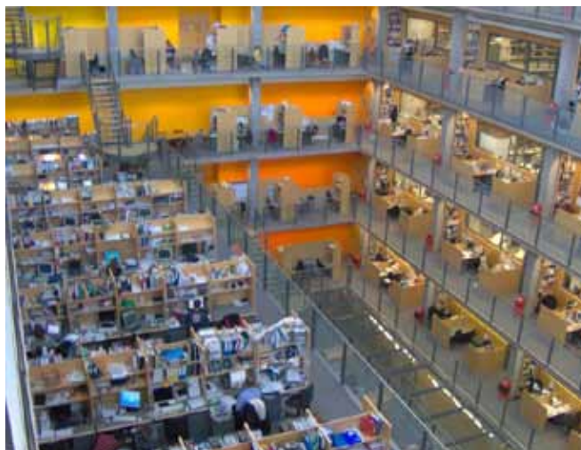
Large atrium with substantial fuel load.
