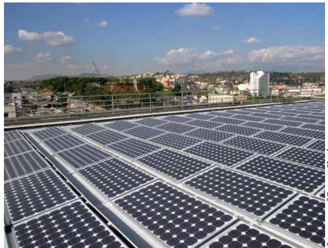
Large PV installation on a warehouse rooftop, effectively preventing any fire dept. roof operations.
