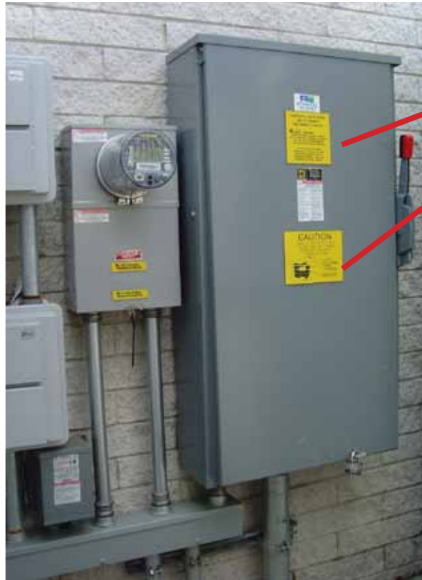
Power Shut-Off for PV System including Inverter
