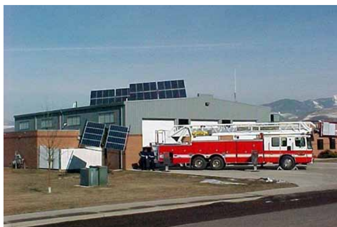
Missoula, Mont. Fire Station with solar power.
