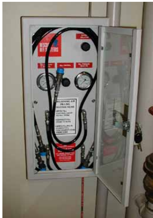
Firefighter breathing air replenishment system
