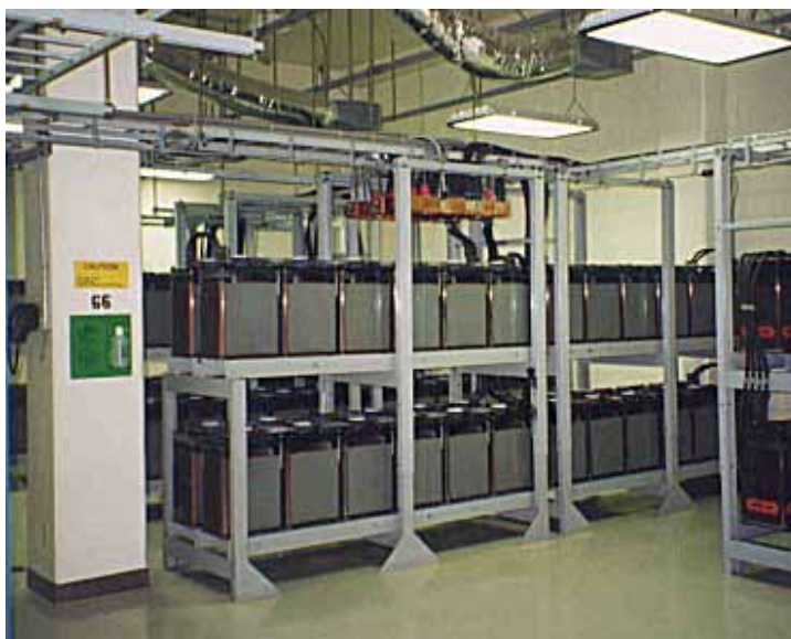
Battery room at a large data center
